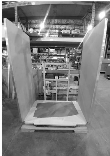
▲ INSTALLED A1 (LEFT) AND C1 (RIGHT) PANELS WITH FINISHING FACING INWARDS
