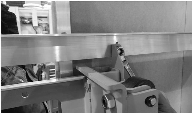
▲ ACCESS EACH HEX BOLT FROM THE T1 INNER PANEL. ENSURE EACH HEX BOLT ON EACH SIDE IS FIRMLY TIGHTENED.
